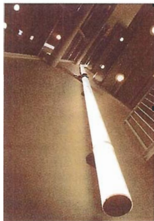
A prismatic light guide makes a Warren Hall's glass-enclosed stairwell a nighttime beacon of light.
